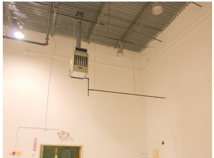
Sample Warehouse Gas Fired Heater
